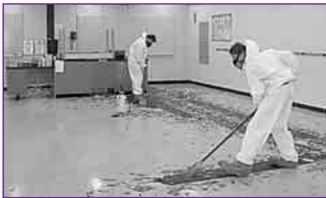
Part of the high school renovation plan called for the removal of asbestos-containing floor tile.
